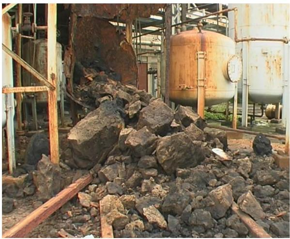
Figure 6. Reaction products spilling from the corroded vessel at the sevin structure. Sample IT02001 was collected from this location. ©Greenpeace/Greig
