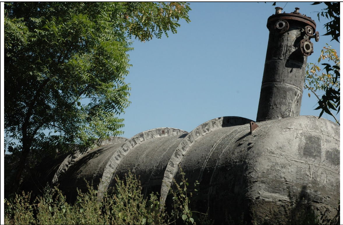
Fig. 4: MIC Storage Tank 610 Side-Head Nozzle Configuration
