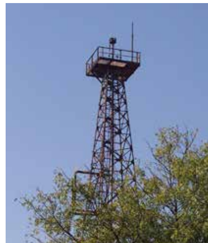
▶ Figure 8. However, the flare was out of service, so the MIC release escaped into the air.
